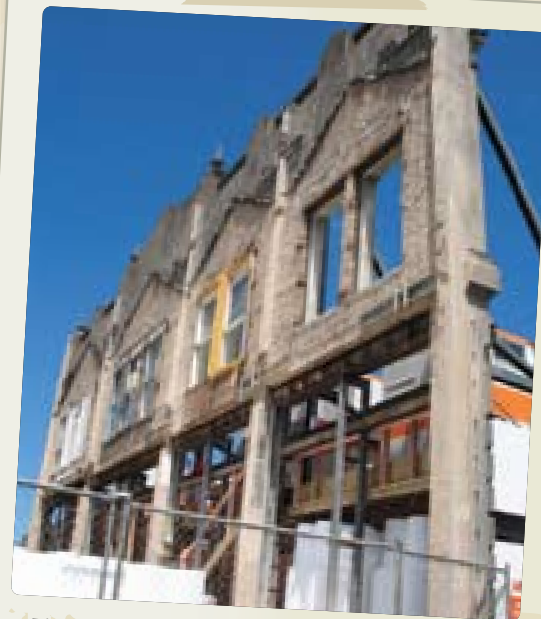
The Chatham Buildings in Central Auckland are prepared for the development of a multi-storey building behind and adjoining. This is an example of façadism.
